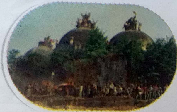
Demolition of Babri Masjid
